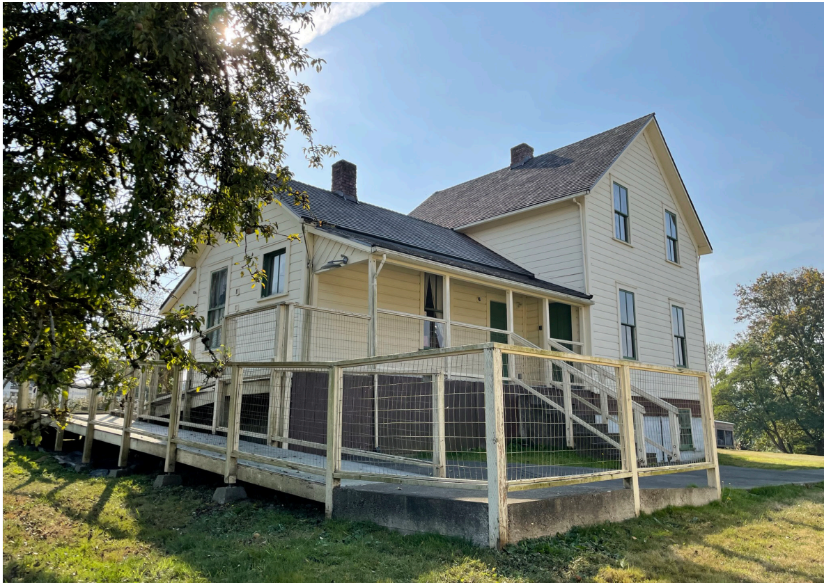
Ramp installed in lieu of the lift, connecting the back porch to sidewalks that lead to the parking area.
