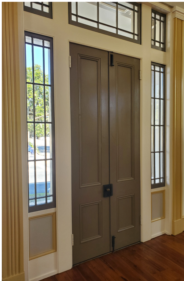
Union Bank of Florida, Tallahassee, Florida. The oldest extant bank in Florida. View of front entrance from interior. Image depicts original wood double doors, which are too heavy for ADA restrictions and do not meet ADA width codes or threshold codes.
