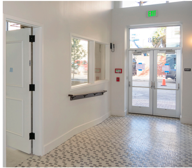
Florida Baptist Building. View of interior facing front entrance, which depicts a re-grade and slope of the interior floor to become flush with the entrance elevation and meeting ADA requirements instead of seeking exemption.
