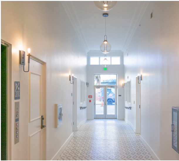
Florida Baptist Building. View of interior facing front entrance, which depicts a re-grade and slope of the interior floor to become flush with the entrance elevation and meeting ADA requirements instead of seeking exemption.
