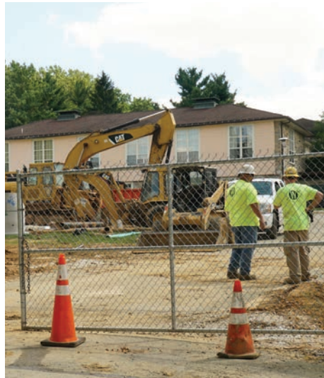
Construction of the new residence hall is progressing smoothly.
