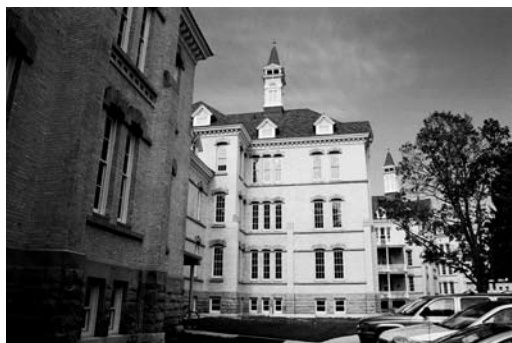
The stepped-back arrangement of the hospital wings allowed rooms to have natural light and ventilation and provided views of the hospital grounds. Pictured here is Traverse City Hospital in Michigan.
