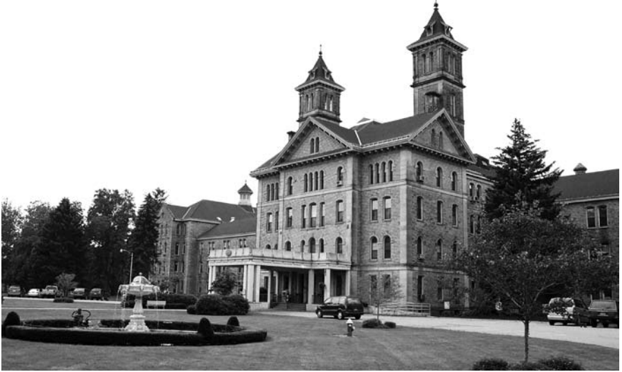
Warren State Hospital (Pa.) has retained its original use, including continuing to provide inpatient health care, but the campus now also houses other health and social services.
